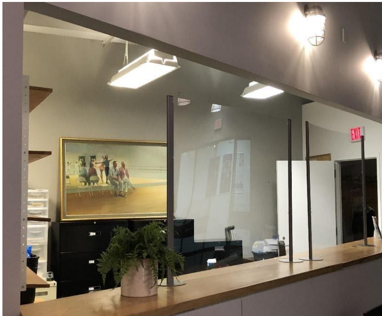
Plexiglass shields have been installed at each front desk location.
